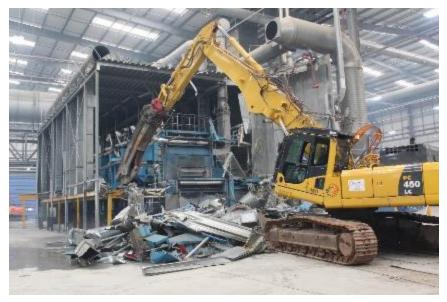
Euro Demolition & Dismantling were appointed to dismantle a number of industrial printing presses and plant as well as carry out demolition works to some of the associated buildings.
